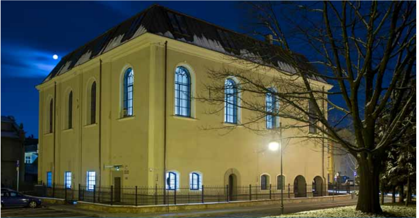
The former Large Synagogue
